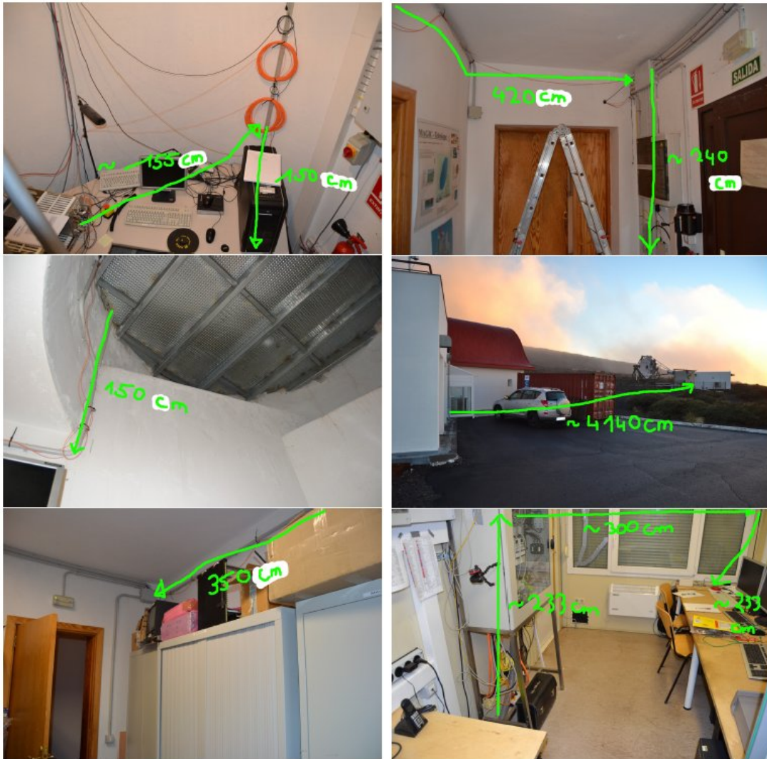
Figure 2.3: The path from the NIM crate to the FTM trigger in board in the FACT container.
